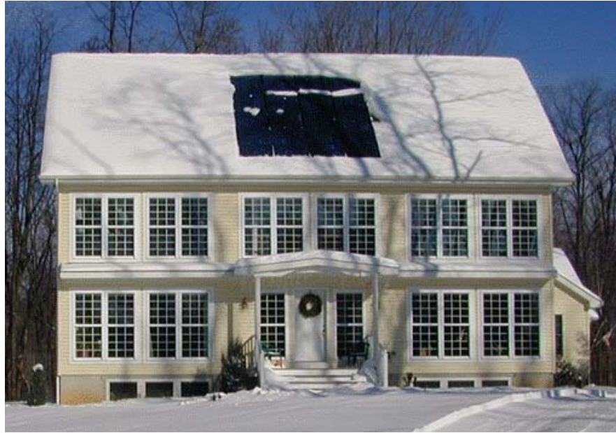
Figure 3: A Passive Solar House in Upstate New York (Photo Richard Perez)
