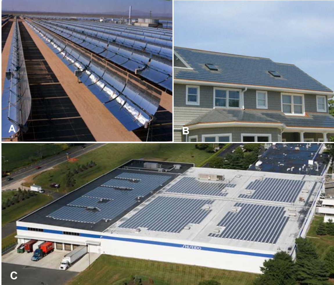
Figure 4: (A) a 100 MW CSP Power plant in Daggett, CA (source NREL PIX Library); (B) a 7 kW residential PV installation (Source AtlantisEnergy); (C) a 700 kW commercial PV installation (Source SunPower)
