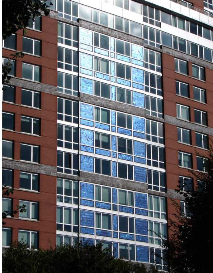
Figure 5: A BIPV Installation in New York City (Photo courtesy of AltPower)
