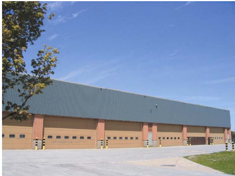
Figure 2: An Industrial Solar Wall Installed at Fort Drum (Photo courtesy of Ron Kamen, Earth Kind Energy)
